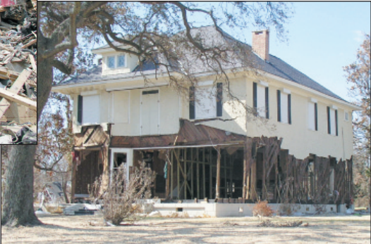
(At right) The main floor of this 2-story house was swept away, leaving the top floor intact but unsteady. Homes near the shore were destroyed. Others have water damage up to three feet high.
